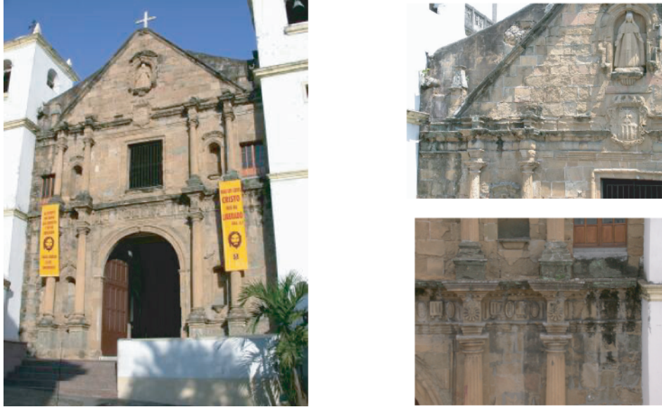
Figure 6.1: The left picture shows Mercede Church, one of the oldest buildings in Panama City. The facade of this church has deteriorated and been cracked by wind and rain, as shown in the right images.
