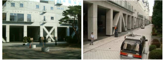
Figure 9: Test scene (photo of our campus building): vertical columns are actually arranged at every 6m.
